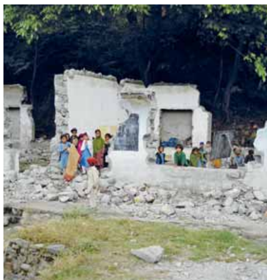
School building demolished by the October 2005 earthquake.
