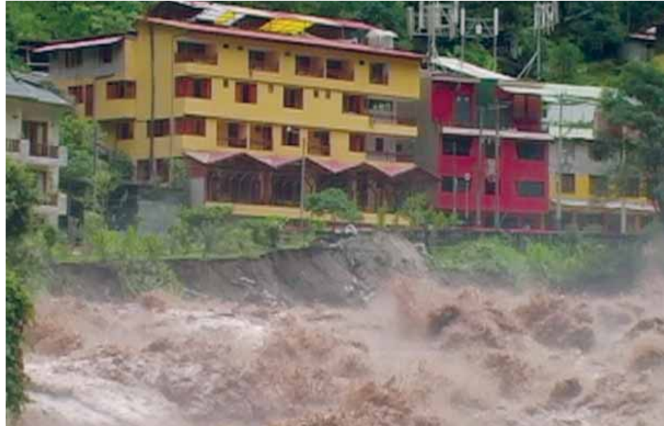
High-cost tourism infrastructure exposed to a mountain torrent Location: Aguas Calientes near Cusco, Perú. Photo credit: La Republica, February 2010
