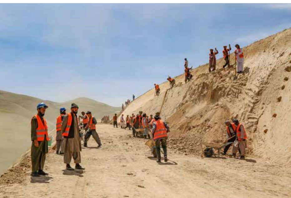
Men work on improving a rural road in Takhar. © SDC
