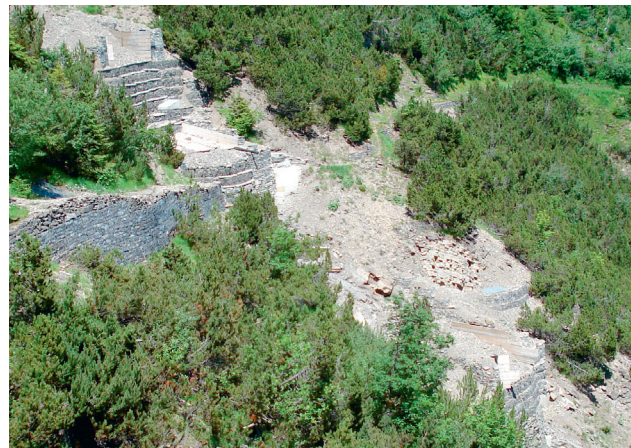
Watershed management using reforestation and slope stabilization (gabion)
